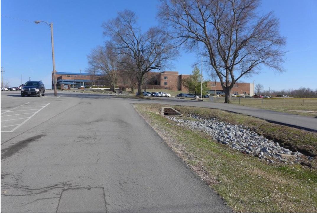
Figure 4-17. Nicholas County High School, Area Disturbed by Construction, Looking N.
